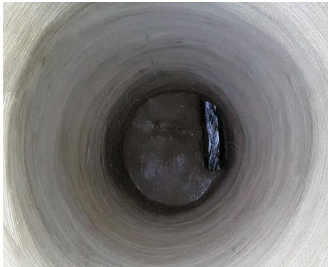
A rehabilitated manhole with a 1-inch-thick coating of MS-10,000, a fine aggregate composite concrete with an anti-microbial admixture.
