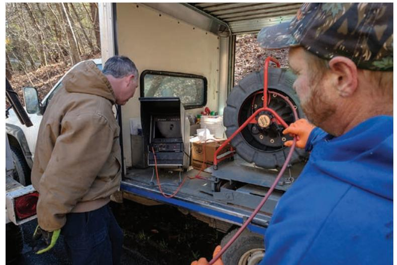
Ronald Miller (left) and Mike Barick keep an eye on the monitor while feeding a camera (RIDGID) into a sewer line for a post-cleaning inspection.
