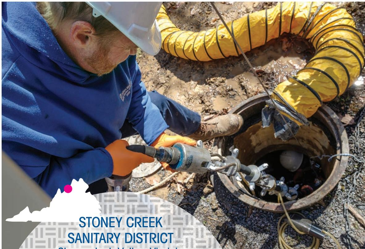
Mike Barick feeds a UV light curing assembly into the manhole where Ronald Miller positions it for the curing operation.
